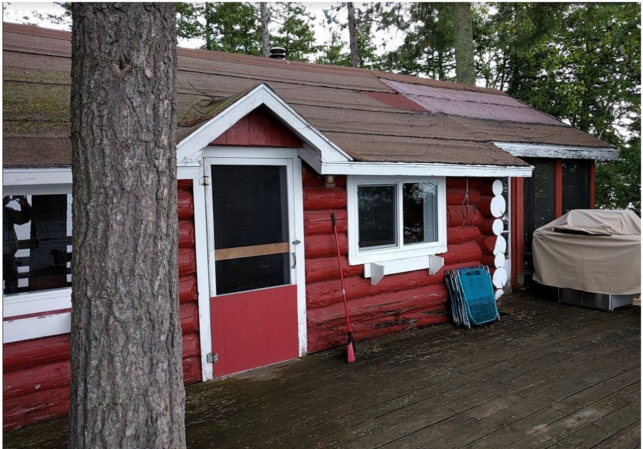
Front of current cabin
